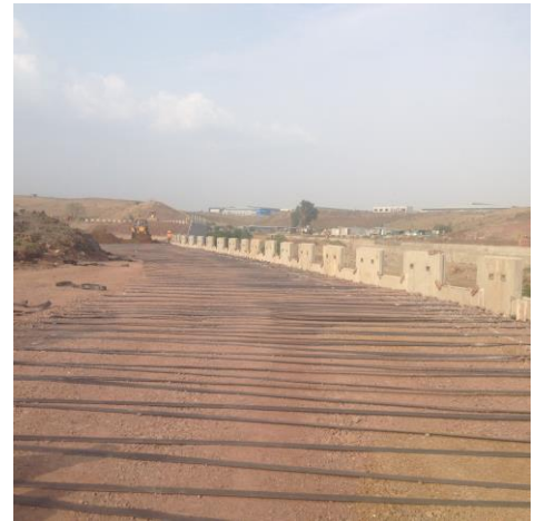
Fig:02 Paraweb laying process
