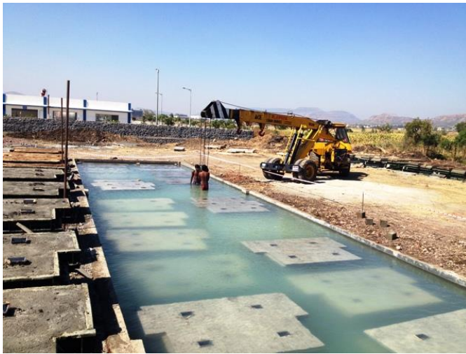
Fig:01 Deep water curing process.
