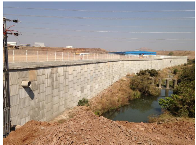
Fig :03 Completed Structure.
