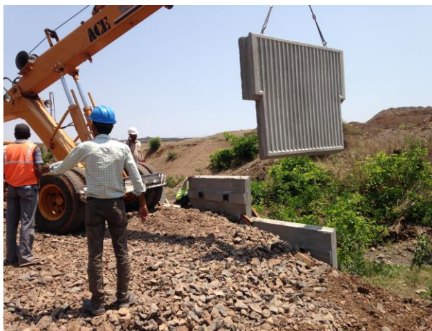
Picture:04 Erection of panel
